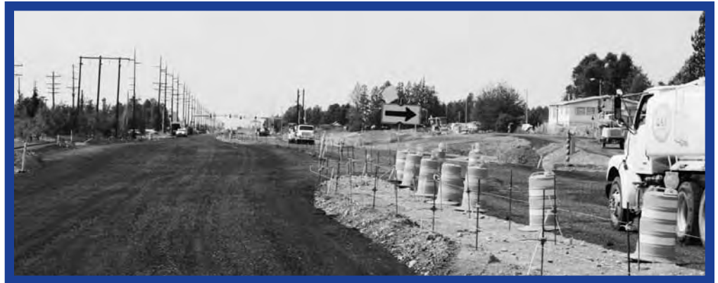
Pictured is QAP's Dowling Road extension project.
