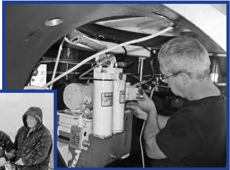
↑ Radar Specialist Jay Fisk is shown hooking up a radar oil system in Cape Newenham.
